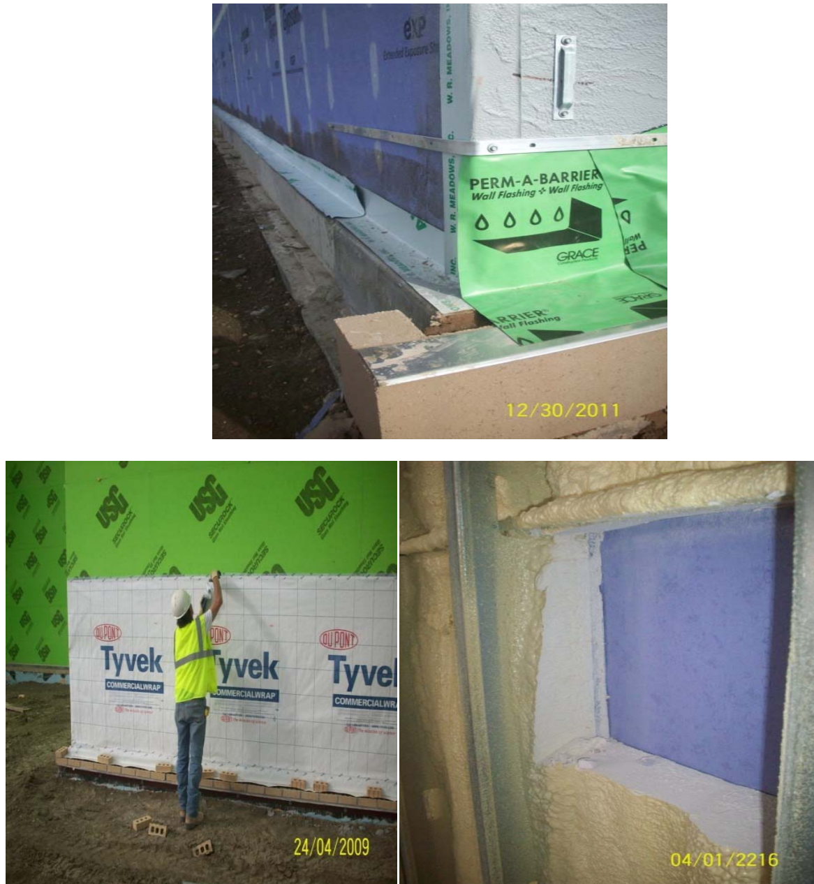
Figure 5: These are examples of the four most common air water and vapor control layer materials. (Top) A fluid applied membrane material and a self adhered membrane functioning as the thru-wall flashing at the mud-sill. (Bottom left) A common mechanically fastened sheet film building wrap product. (Bottom Right) A cut out section of a closed cell spray applied foam applied to the interior cavity of the exterior wall assembly.
