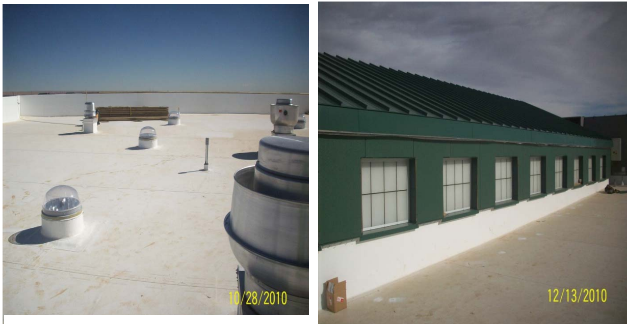
Figure 1. – Left is an example of a fully adhered TPO membrane roof system. On the right, a standing seam metal roofing system.
